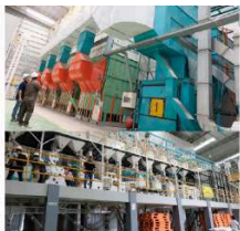
MODERN RICE MILLING PLANT
